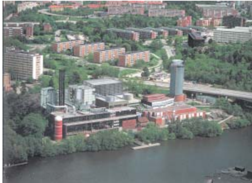
Solna heat plant with the new fuel handling and flue gas cleaning system. Photomontage: Scheiwiller Svensson Arkitektbyrå.
