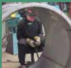
Part for the new pellets plant on the way to be properly installed.
