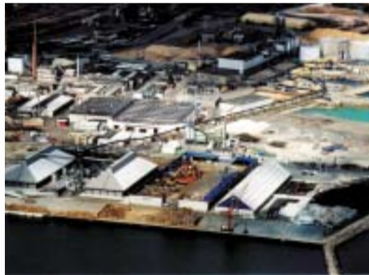
Seen from the harbour with the 700 meters conveyor connecting the production plant with the storage of the ready made pellets.
