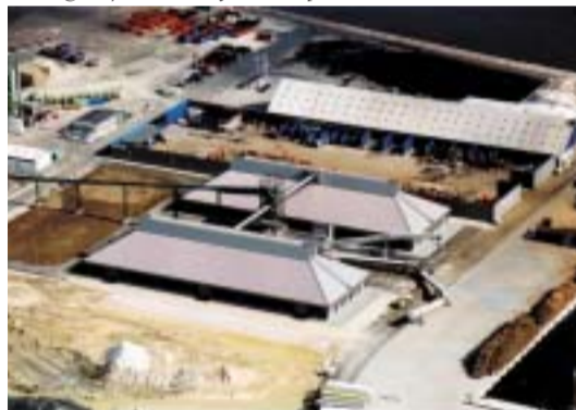
Storage of pellets before shipping to the users.
