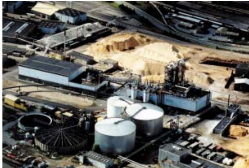
The pellet plant in Køge with the straw storage to the left.
