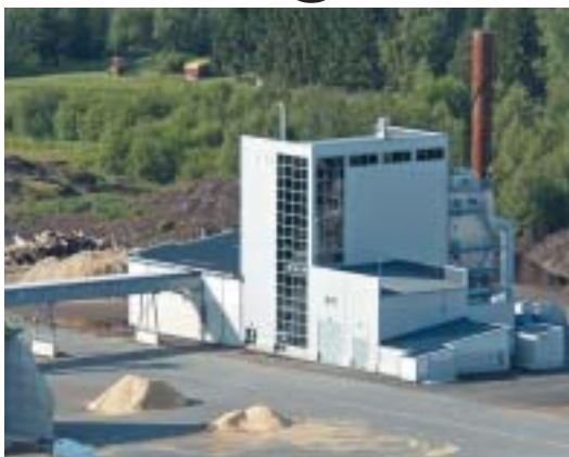
The plant at Renko in southern Finland.
