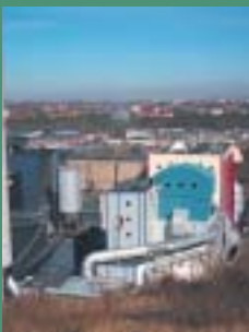
The Högdalen plant in Stockholm features a 91 MWth CFB unit burning sorted commercial waste.
