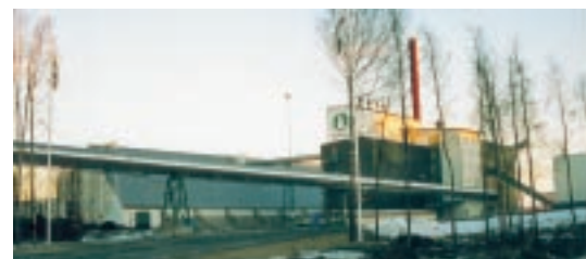
The pipe with the drying gases with the pelletsplant and storage facilities in background.
